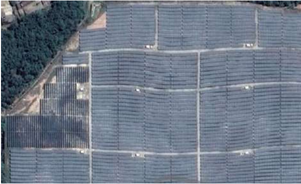
Figure 3-7 PV plant panoramas
