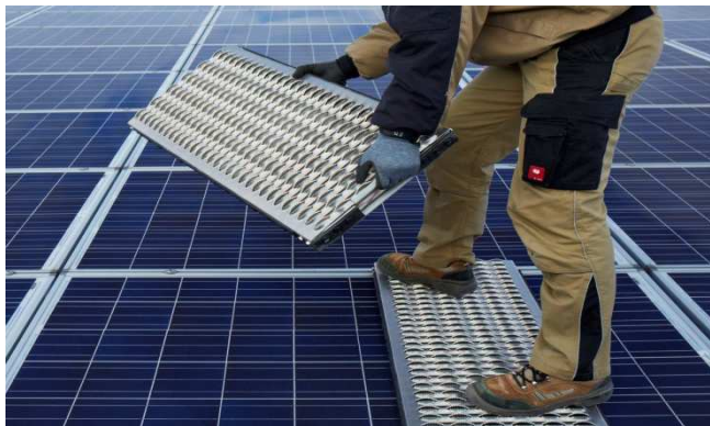
Figure 7: Placing the SMB SOLAR MULTIBOARDS®
