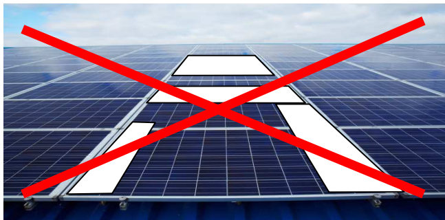
Figure 4: Incorrect alignment of SMB SOLAR MULTIBOARDS®
