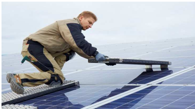
Figure 8: Inserting the SMB SOLAR MULTIBOARD®
