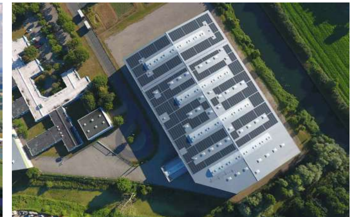
KLEVE, GERMANY 749 kWp
