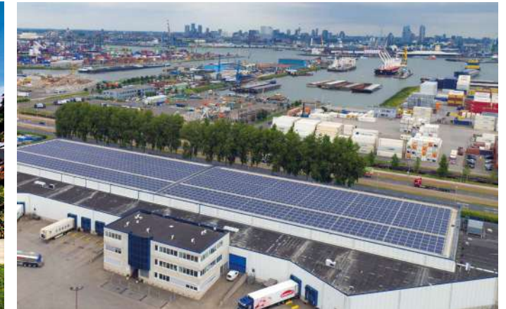
ROTTERDAM, NETHERLANDS 822 kWp
