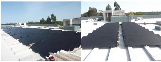
One of the most recent and advance private hospitals in Portugal choose a Energie thermodynamic solar system to provide all of their DHW and large savings. Was installed 4xEco6000 with AISI316 stainless steel cylinders, with a total of 160 solar panels.
