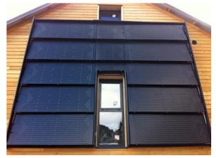
A skier's refuge at 1800m altitude at the Pyrenees. A special model Eco1500 for DHW with 10 solar panels was designed for this specific solution. An excellent architectural integration. The DHW is used for the rooms and restaurant.
