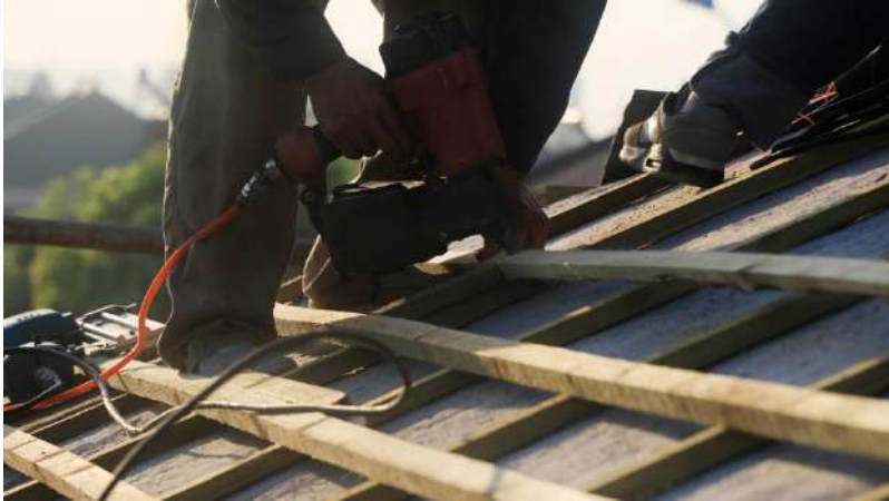
Install water strips and hang tiles
