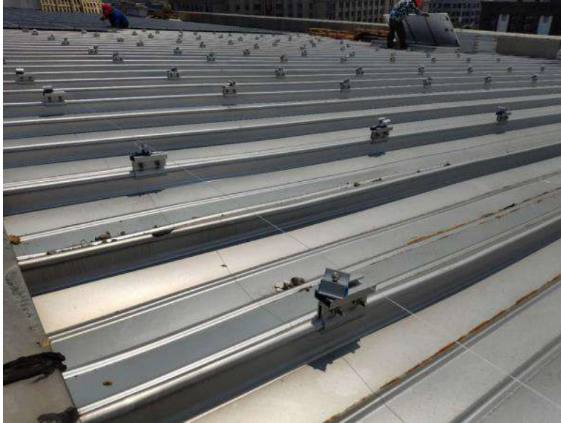
Install roof hook
