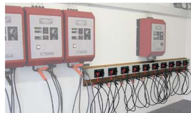
Example for Steca BAS (battery connection system)
