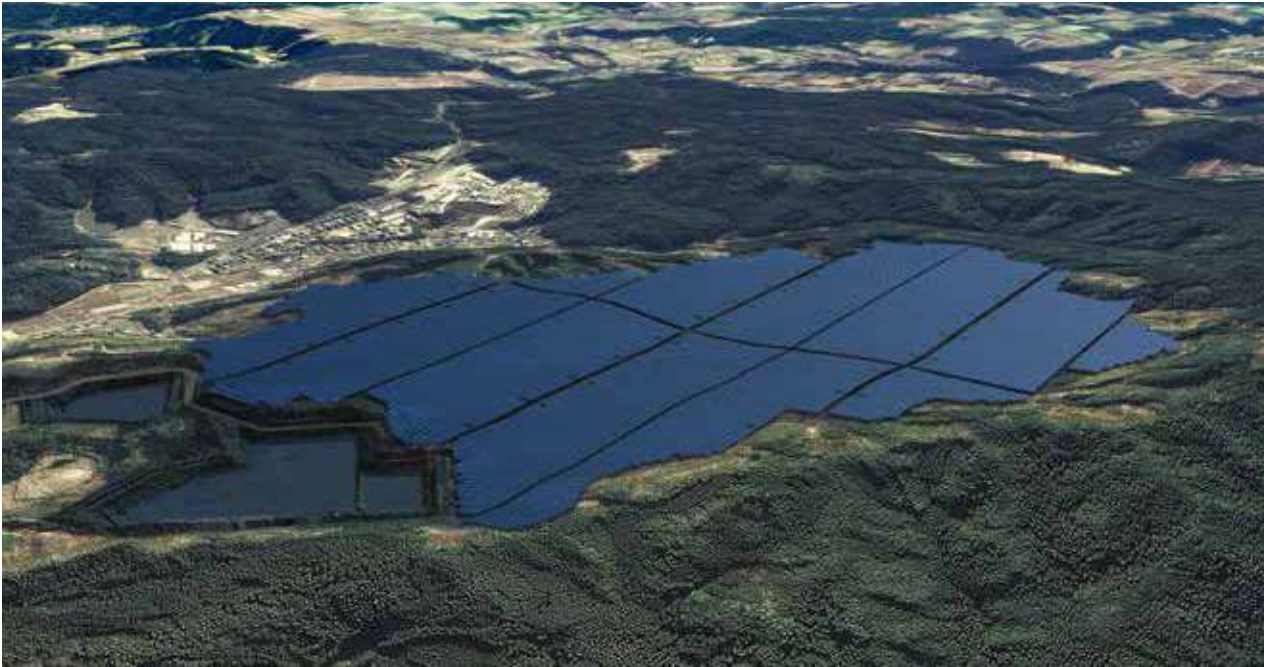
Miyazaki City, Miyazaki Prefecture, Japan 96.2MW / Tallmax / 2018
